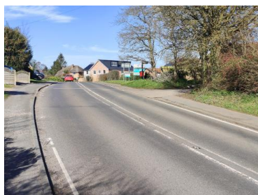
Approaching from the South
